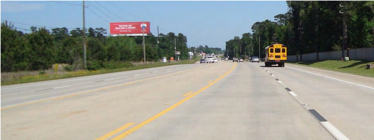
Figure 2.3: FM 1488 Existing Roadway
